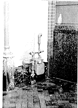
Utilities should not be exposed at the sidewalk because they run the risk of damage.
