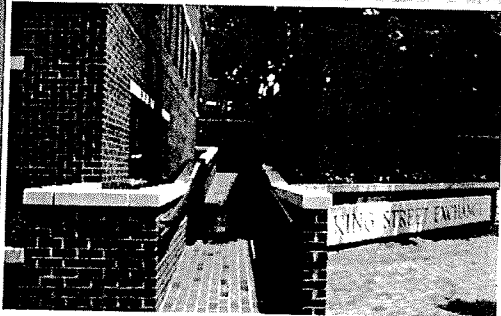
This design provides universal accessibility as a site feature, well integrated with the landscaping and able to easily accommodate signage.
