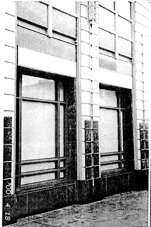
A three-part ordering of the building face is achieved at grade with the careful application of building finishes. Note the greater sense of weight the darker finishes provide at the base.
