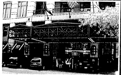
A building canopy can serve as a visual amenity as well as shelter for building occupants and pedestrians.
